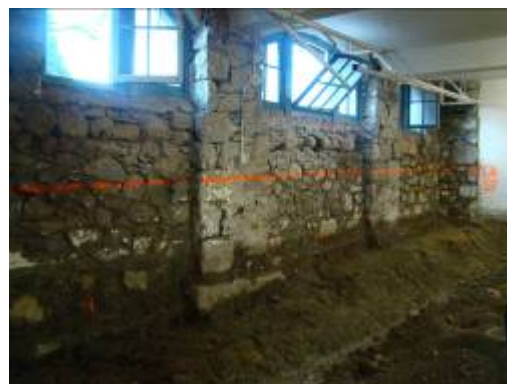
Excavation of the original foundation wall
